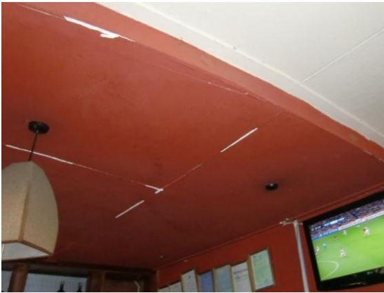
Figure 21: Ageing ceiling with cracks
