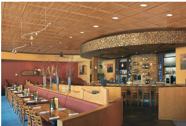
Figure 43: Sample ceiling from recycled wood
