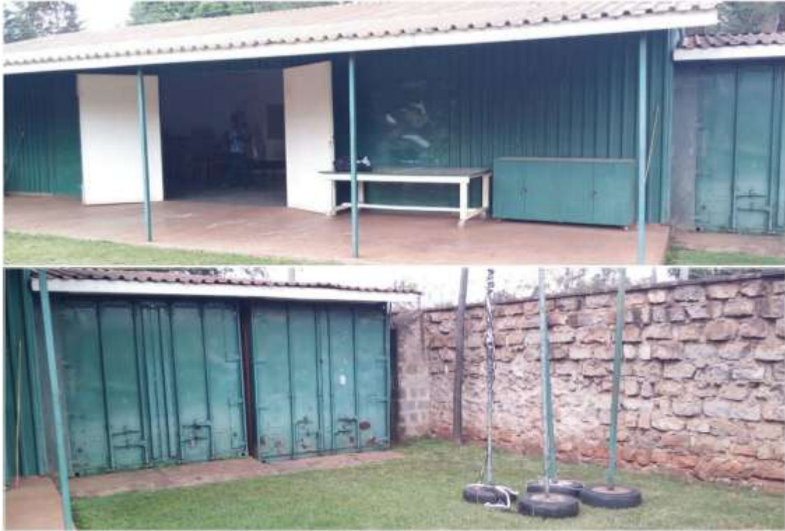
Figure 8: View from the front of the structure
