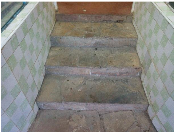
Figure 4-23: steps at the main entrance. Source: (Author, 2020)
