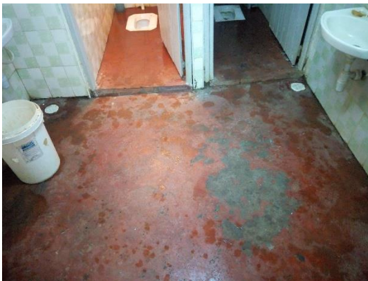
Figure 4-21: worn out cement on the floor. Source: (Author, 2020)
