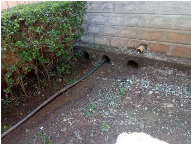
Figure 4-7: water drainage pipe. Source: (Author, 2020)
