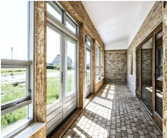
Figure 2-31: wall covered with OSB panels
