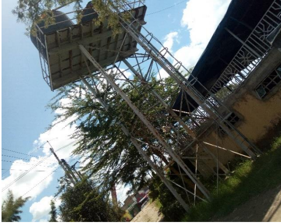
Figure 4-8: water tower and tanks. Source: (Author, 2020)
