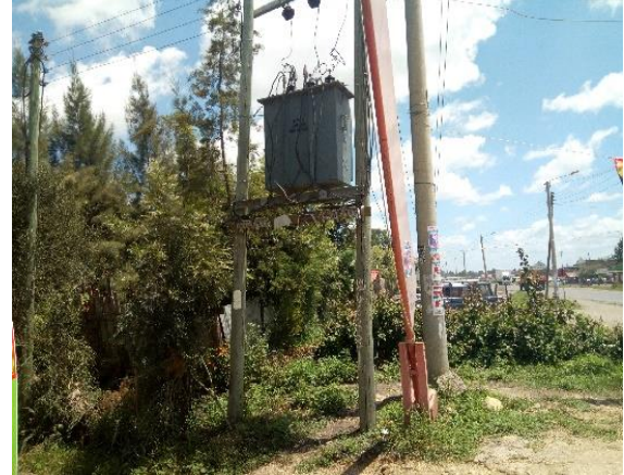
Figure 4-9: electricity transformer. Source; (Author, 2020)
