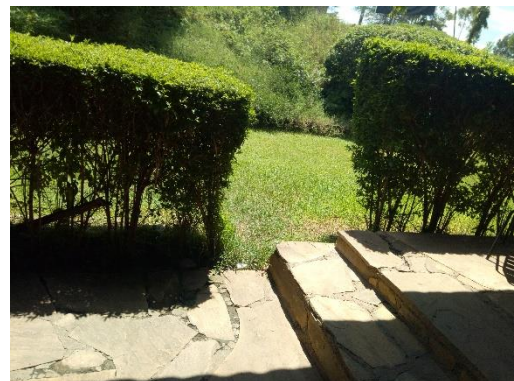
Figure 4-10: steps with mazeras floor finish. Source: (Author, 2020)
