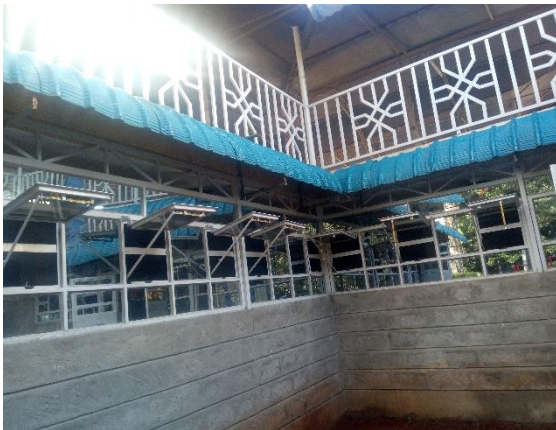
Figure 4-17: window openings. Source: (Author, 2020)
