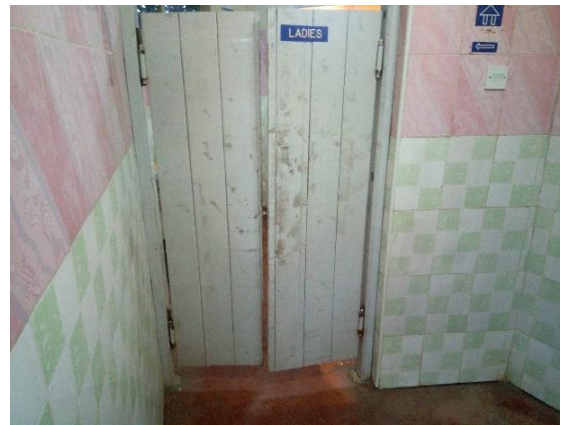
Figure 4-22: wooden double door. Source: (Author, 2020)
