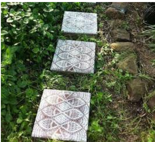
Figure 5-26; stenciled concrete on walkway. Source: (Noonan, n.d.)
