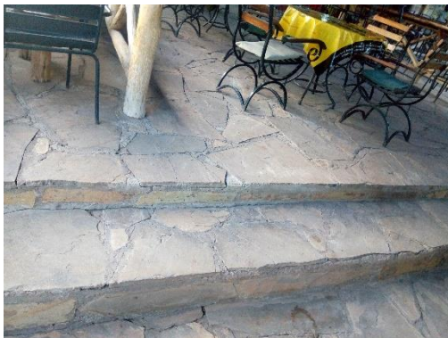
Figure 4-11: mazeras floor finish. Source: (Author, 2020)
