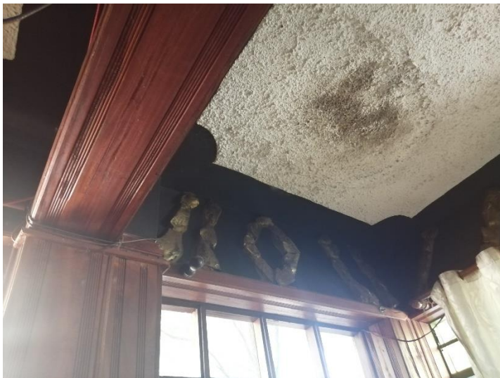
Figure 4.20: White stucco ceiling (Source: Abbas, 2019).
