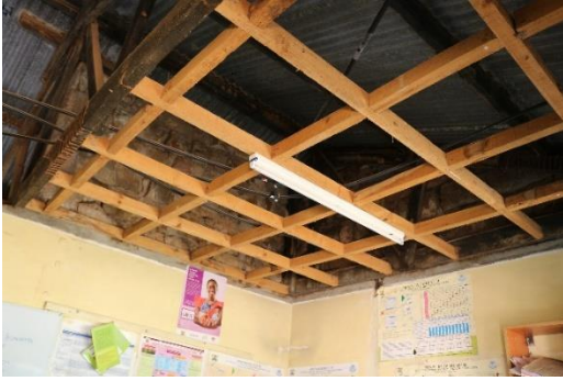
Fig 4.1.8 Exposed ceiling trusses (source, author2019)
