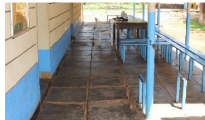
Fig 4.2.1 worn out floor (source author, 2019)
