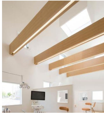
Fig 5.0.2 Wooden ceiling beams with inbuilt lights (source google.com)
