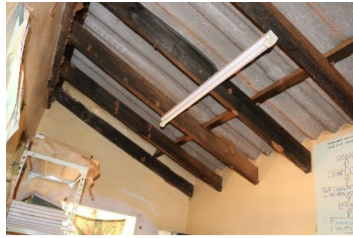
Fig 4.1.9 Asbestos ceiling (source, author2019)
