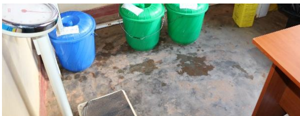
Fig 4.2.0 Simple cement floor (source author, 2019)
