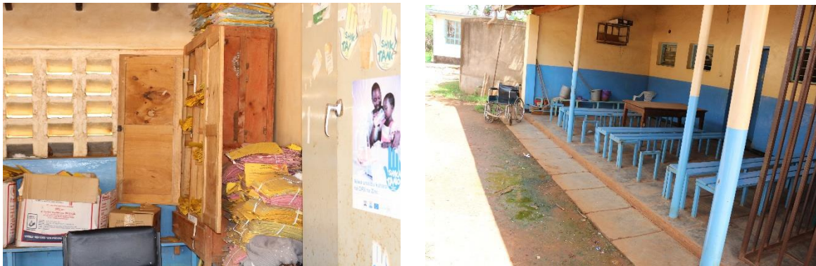
Fig 4.2.9 Cabinets on the wall (source author 2019) Fig 4.3.0 waiting area (source author 2019)
