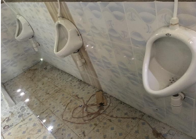
Figure 4.15 Washroom area (Source: Author, 2020).
