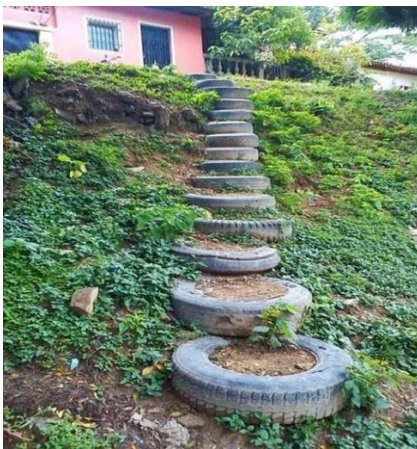
Figure 2.16 recycling tires for yard landscaping steps
