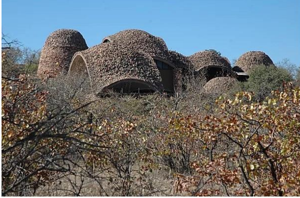
Fig. 2. 10 Fig. 10 Mapungubwe National Park, Source: (PETER RICH ARCHITECTS, 2018)
