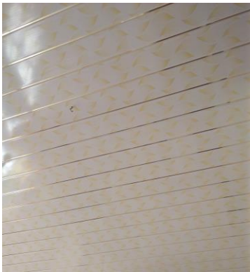
Fig. 4. 6 Yoeligen hotel vinyl ceiling, Source: (Author, 2019)
