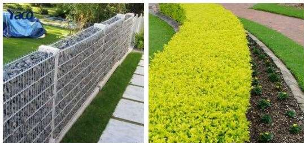
Figure 24: Gabion wall and hedge fence (Source, Pinterest, 2020)
