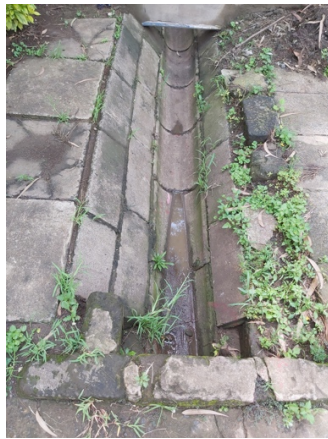
Image 23: Open storm water drainage
