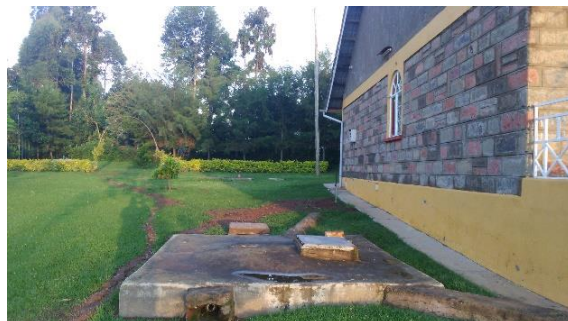
Figure 4.37 Outside underground reserve tank (Source; Camera author)
