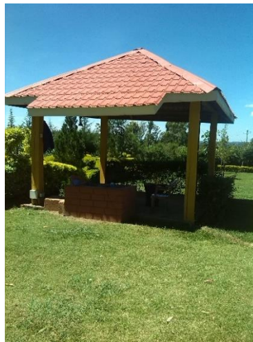
Figure 4.42 Patio (Source; Camera author)
