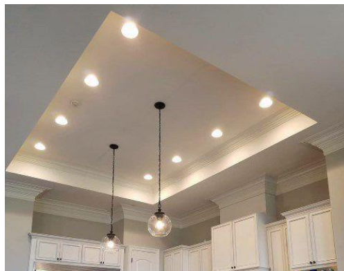
Figure 5.27 recessed Gypsum ceiling (Source; Pinterest.com)
