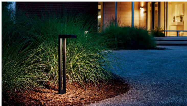
Figure 5.19 Ground lighting (Source; Google Images)
