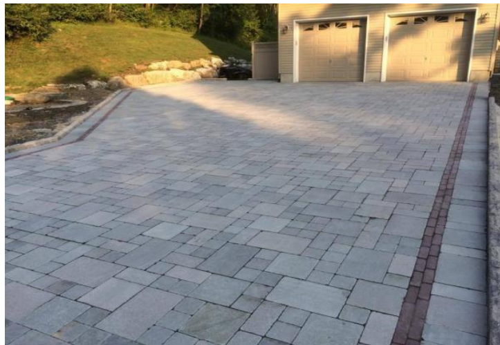
Figure 5.7: parking lot with cabros Source: hpdconsult.com
