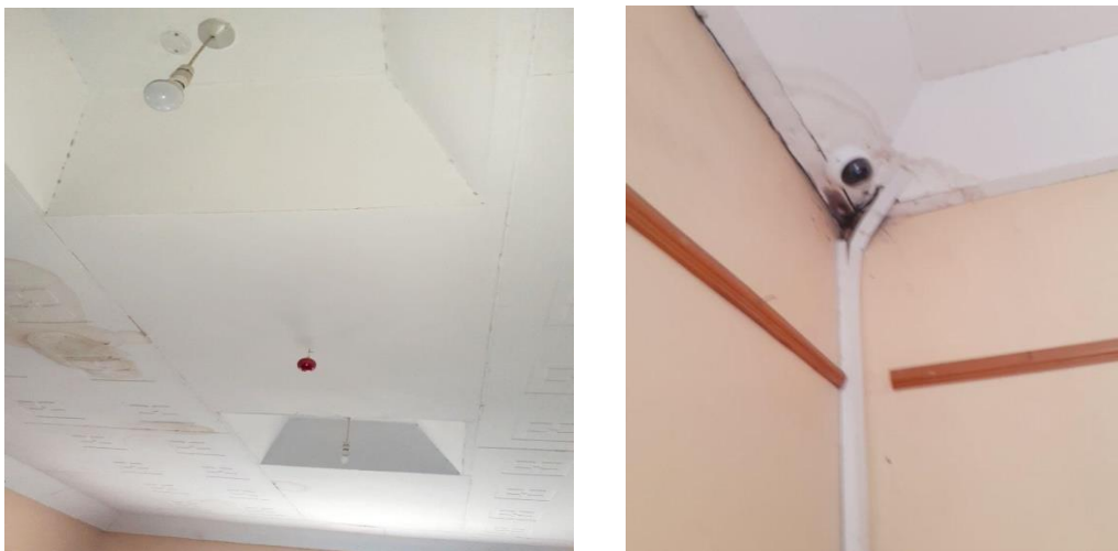
Figure 4.13: Stained MDF ceiling and MDF cornice respectively (Source: Author, 2019)
