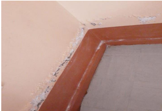
Figure 4.14: Edges of flacking walls and concrete skirting (Source: Author, 2019)
