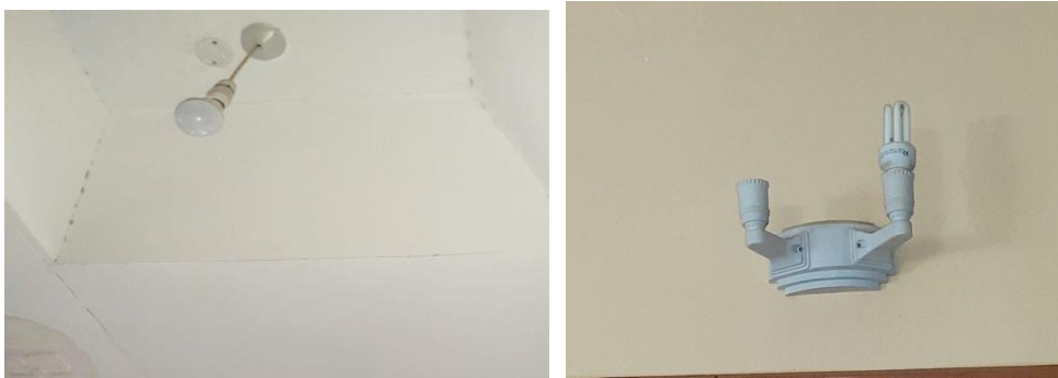
Figure 4.16: Incandescent bulbs on the ceiling and wall respectively (Source: Author, 2019)
