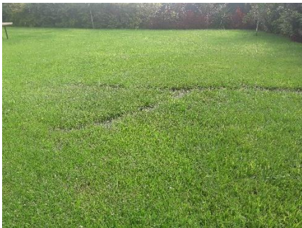
Figure 4.26: Forked drainage trench at the southside of the garden.(Author,2020)
