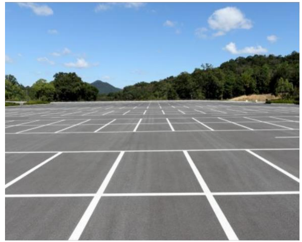
Figure 5.26:Asphalt on parking
