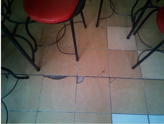
Figure 4.2.1: Worn out ceramic tiles
